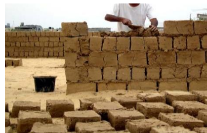
Fig. 8: Construction with mud Blocks (Source- bachillerato-virtual.org )
