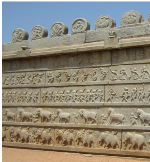
Fig. 14: Wall of temple constructed by using prefabricated stone Slabs.
