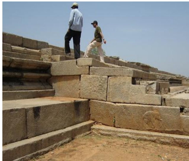
Figure15: Prefabricated stone blocks used to build steps.
